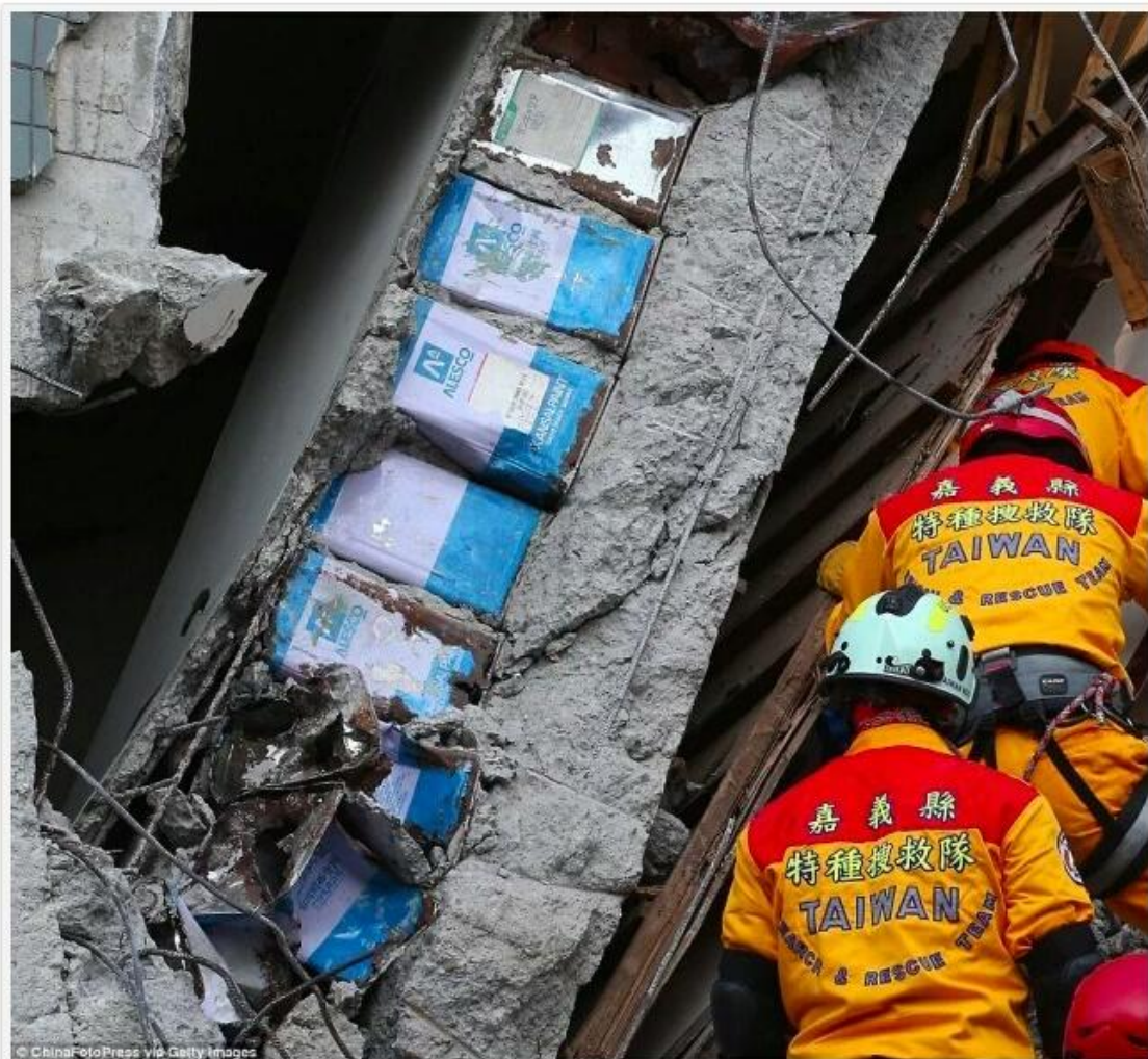
Tin cans within the structural columns in the Weiguan Jinlong apartment complex in Taiwan (via China Foto Press)
